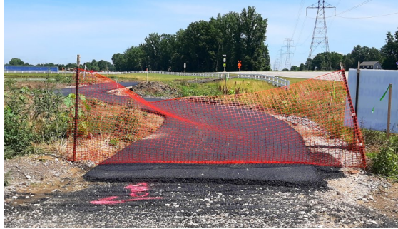
A multi-use path during construction near Olentangy Berlin High School
