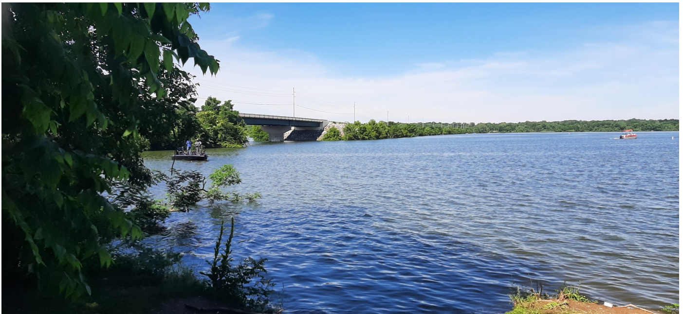
Alum Creek Reservoir and the Cheshire Road bridge
